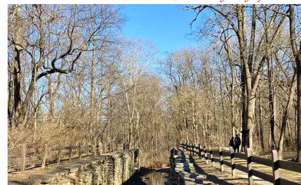
Photo of Lock 12 of the Susquehanna and Tidewater Canal, c. 1836-1855, courtesy Heritage Strategies, LLC
