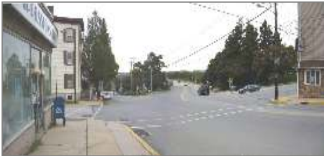
Where Hellam St., Second St. and the bridge entrance come together is unsafe for pedestrians and can be confusing to drivers.
