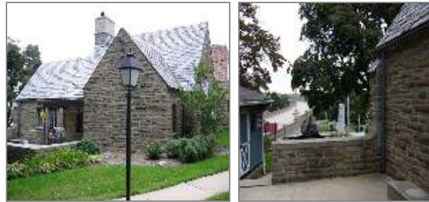
To the south of Veterans Memorial Bridge in Wrightsville is the original bridge administration building, which might someday become a visitor center.
