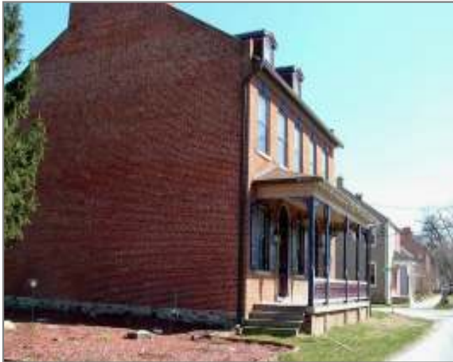
Washington Boro has had a longstanding relationship to the river, evidenced by the character and layout of its existing buildings.
