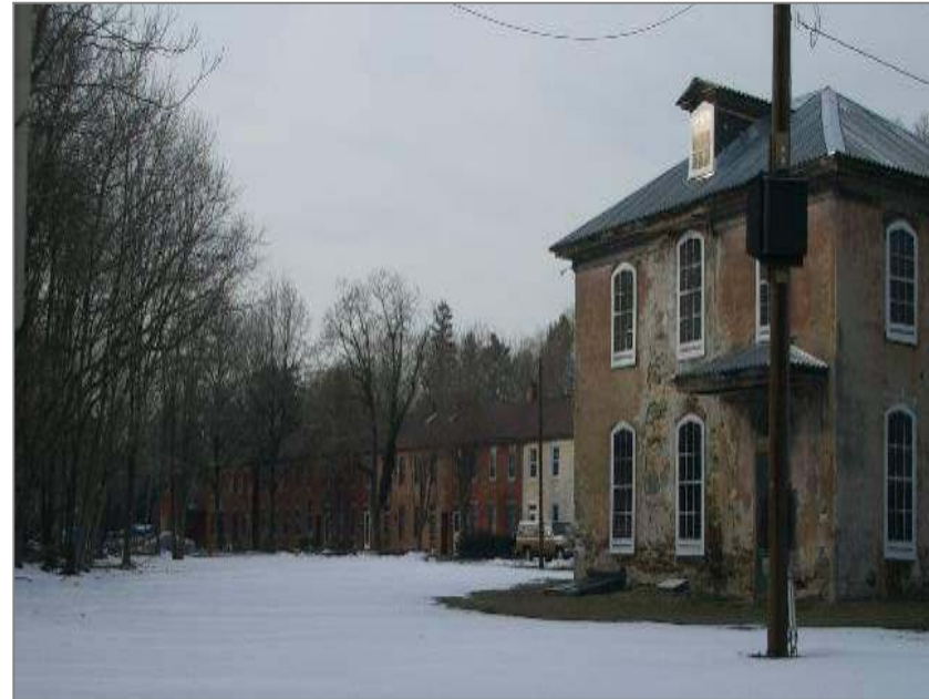
The Vesta Furnace site includes the furnace's historic office building and worker housing.
